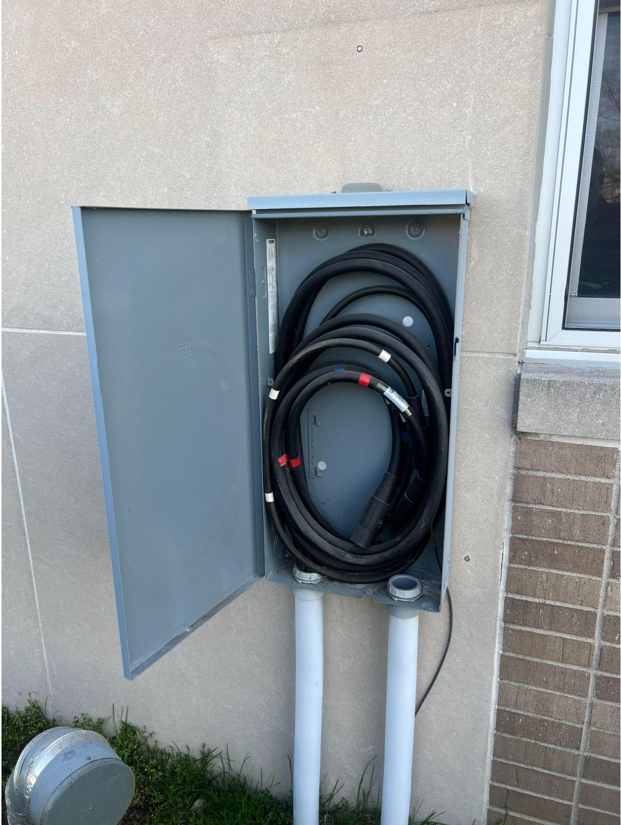
Example of External Generator Connection
